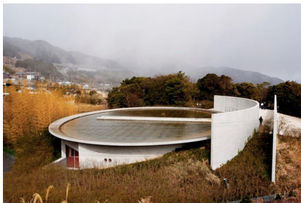
Fig. 9. The Hompukuji Water Temple, Japan
